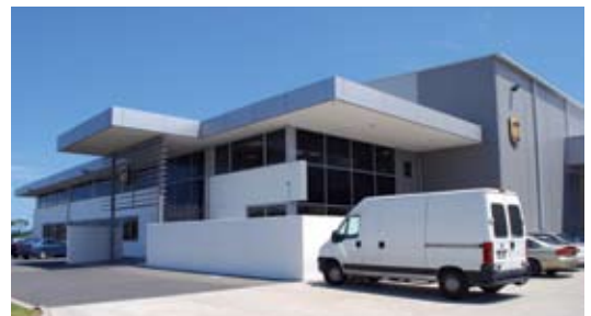
UPS SCS (NZ) Ltd, Pavilion Drive 8400 2 Office/Warehouse/Canopy
