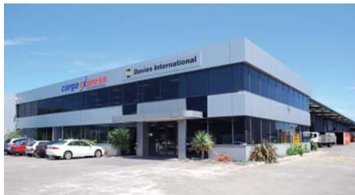
The drive-through complex for Davies International Freight with entrance on Montgomerie Rd and exit in Aintree Ave 5200m 2 Office/Warehouse/Canopy
