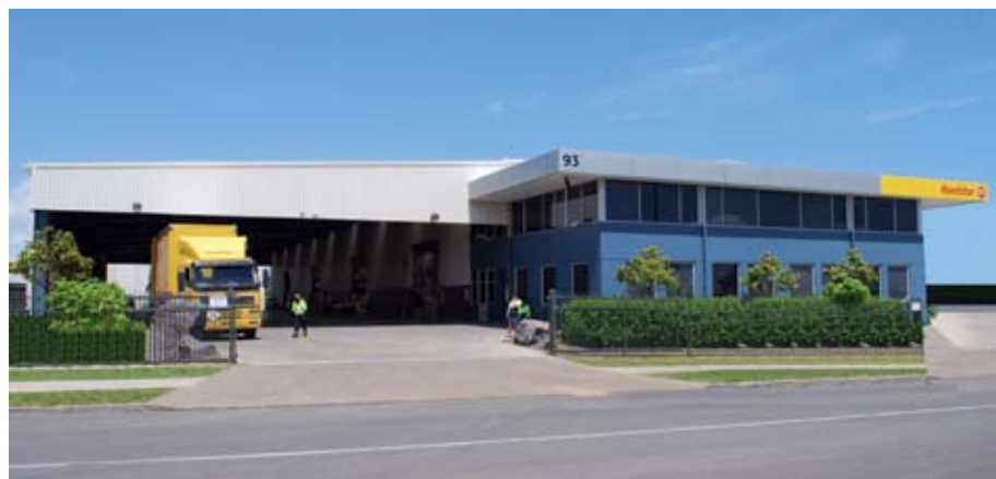
Roadstar Transport Ltd, Airpark Business Centre, Auckland
